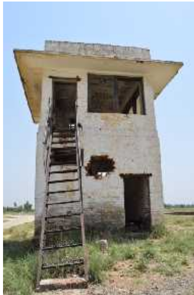
Plate.3 Signal Cabin. Doors, Windows, Ventilators and Stairs.
