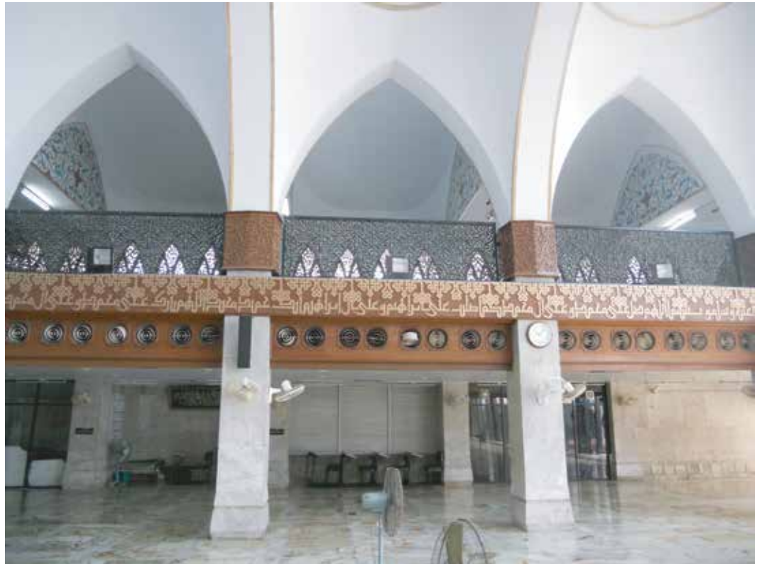
Plate 18. The arcade with equilateral arches and square base piers supports the Women's Gallery on the northern side.
