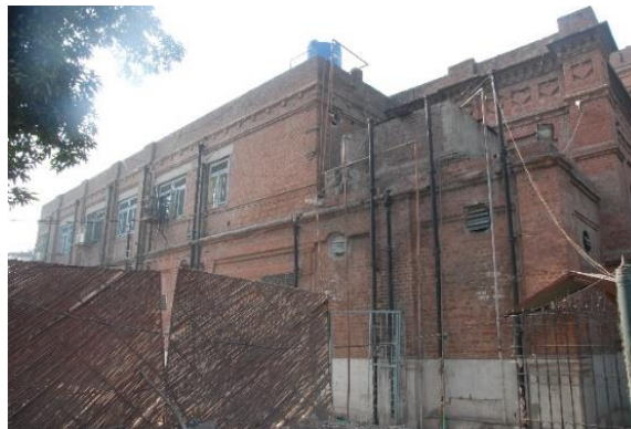
Figure 16 Abnormal Addition on Eastern Side
