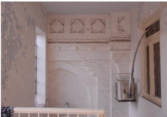
Figure 15 Defacing of Architecture
