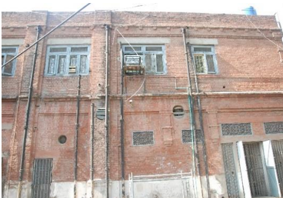
Figure 17 Deterioration of Structure
