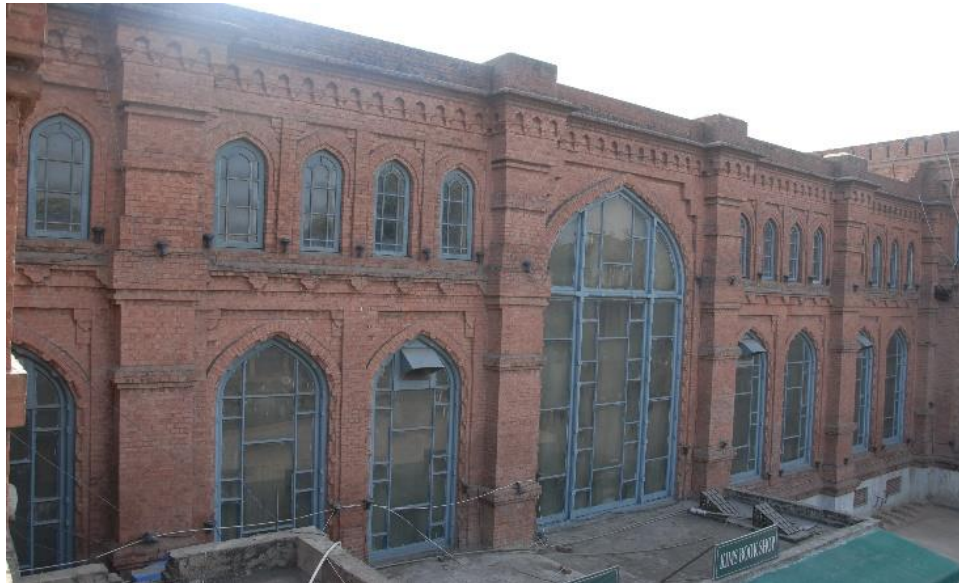
Figure 11 Wing Between Main Entrance and Western End Gallery
