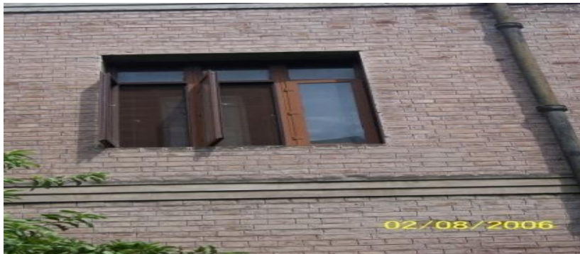
Figure 22- Outer Look of Extension New Building
