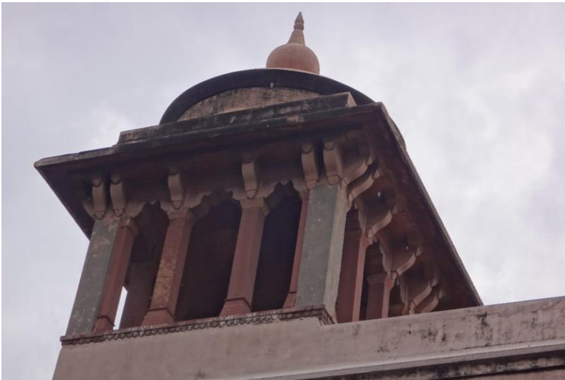
Figure 7- View of Arched Pavilion
