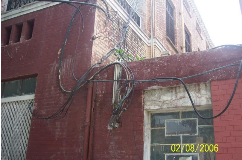
Figure 17– Outer Portion of the Main Building
