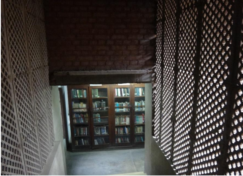
Figure 20– Jālī work of the Main Building.
