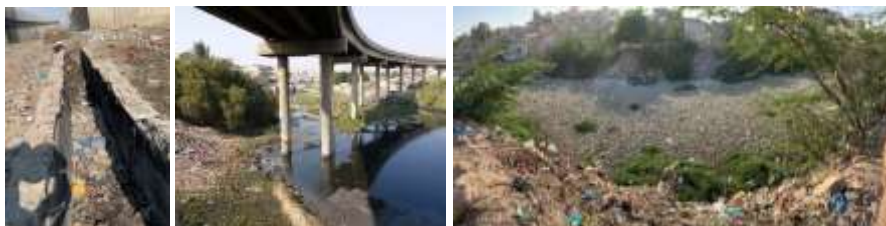
Fig. 33. Open sewer drain
