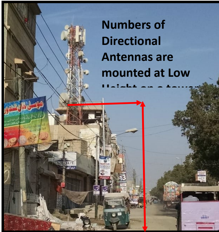
Figure 11: Low heights antennas
