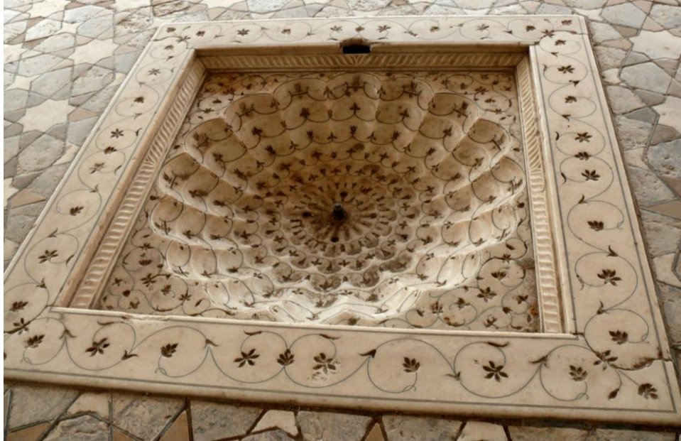
Figure 13. Pietra-dura on Floor of an Indoor Marble Fountain, Lahore Fort
