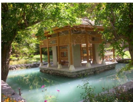
Plate 17. Baradari or pavilion in the Shigar Fort Complex in Mughal Period
