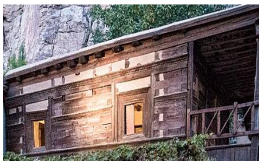
Plate 8. Eastern wall of the Old Resident House adjacent to the main entrance of the complex, with dhajji diwari and window with woodcarving.
