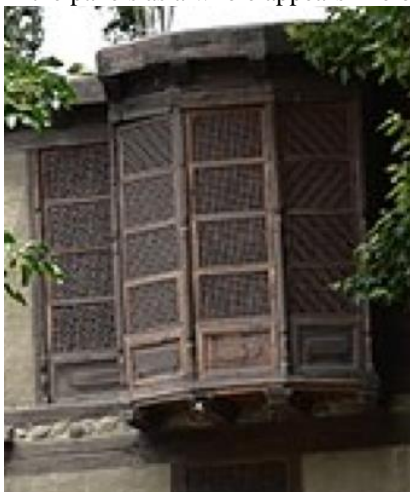
Plate 11. Balcony with mashrabiya screens on the South wall of the Fort
