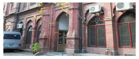
Interventions: AC out-door units, electric ducts, electric DB, paint on wooden railing, electric cables, fiber glass shed, Security grills, paint on wood, Spot lights
