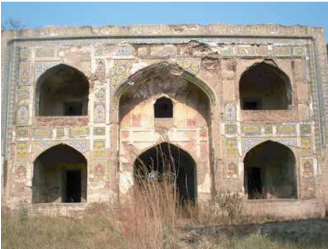
Plate 3. Rear façade of the gateway to the Tomb of Ali Mardan Khan, facing south.
