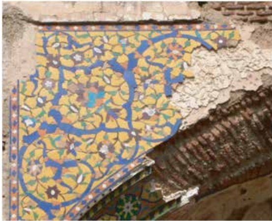
Plate 16. Islimi-khata'i on the spandrels of the central arch of the gateway
