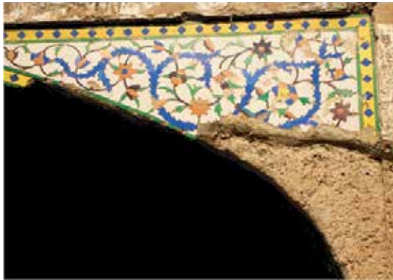
Plate 17. Faience mosaic from the lower side arches of the south façade of the gateway of Ali Mardan Khan's tomb.
