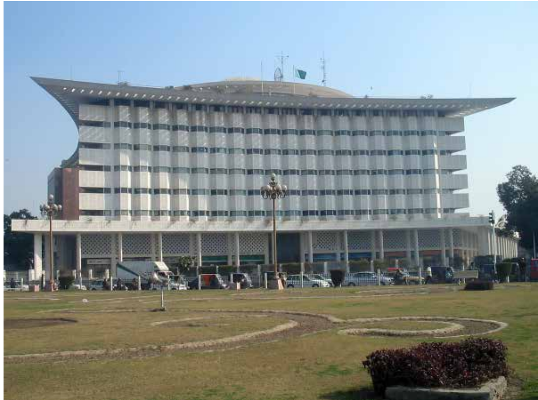
Figure 3. WAPDA House, Lahore. Edward Durrell Stone, architect.
