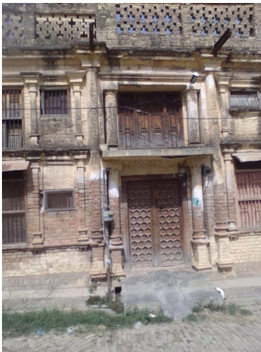
Fig. 22, A house near bus stop of Bhoun
