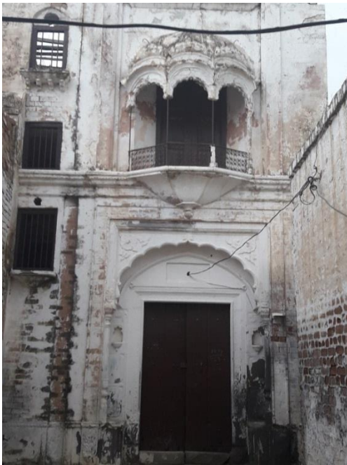
Fig.18, An entrance of haveli in main bazaar
