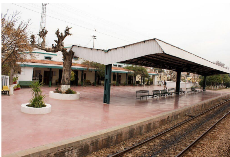
Fig.4.Chaklala Railway Station Track
