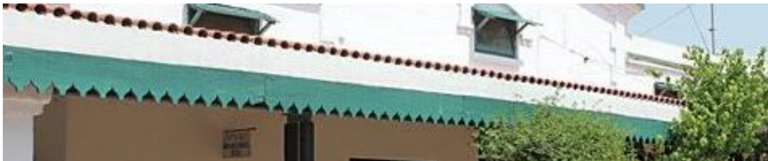
Fig.06. Wooden fringe on the Façade of the Chaklala Railway Station
