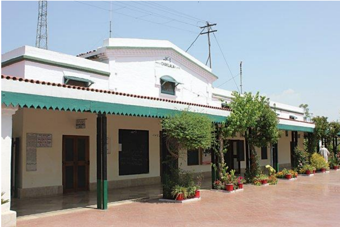
Fig.05. Building of Chaklala Railway Station
