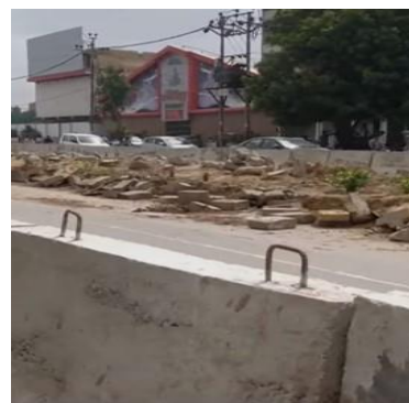
Fig. 10 Construction condition along the route
