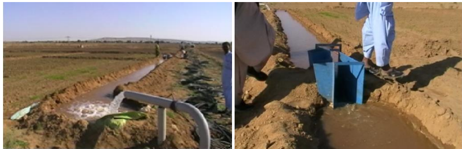
Picture 1. Measuring Discharge through cut-throat flume
