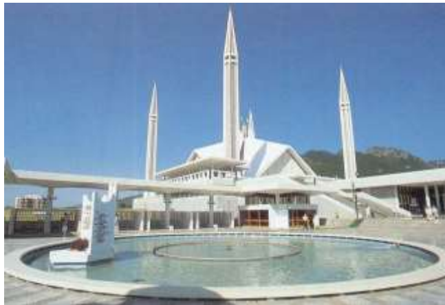
Figure 2. South entrance of the Faisal Mosque Islamabad.
