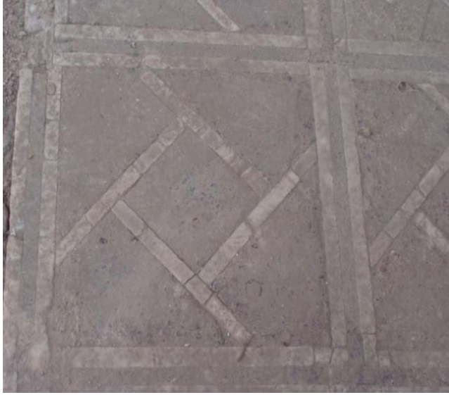
5. Floor, dressing room Shahjahani Hammam,Lhr Fort
