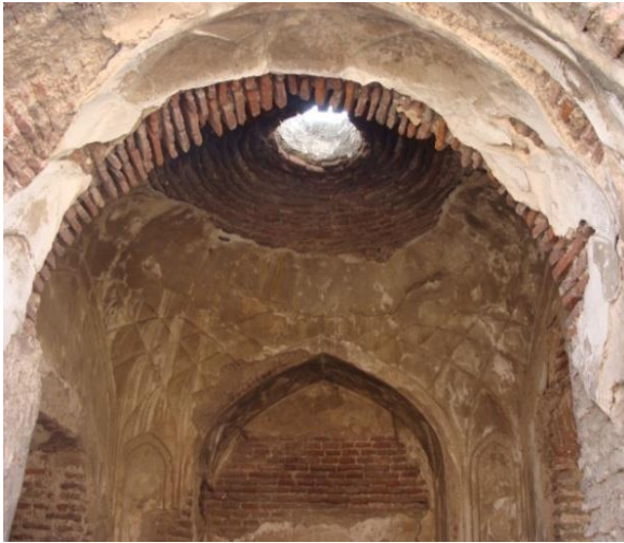
15. Interior, Central Chamber, Ladies Hammam, Lahore Fort
