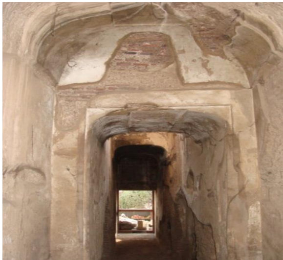
11. Passage opening towards South, Shahjahani Hammam, Lahore Fort
