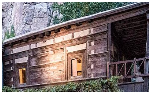
Plate 8. Eastern wall of the Old Resident House adjacent to the main entrance of the complex, with dhajji diwari and window with woodcarving.
