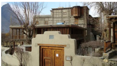
Plate 2. Imposing view of the Shigar Fort Complex House of the complex.
