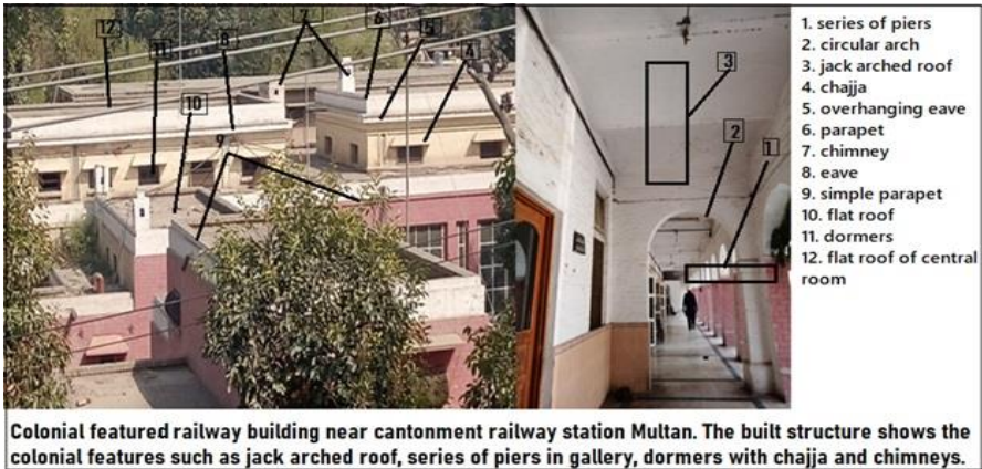
Figure R5: Railway built structure with colonial feature near Cantonment railway station Multan.
