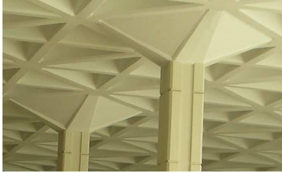
Figure 3. Capitals of the square piers in the ablution area.
