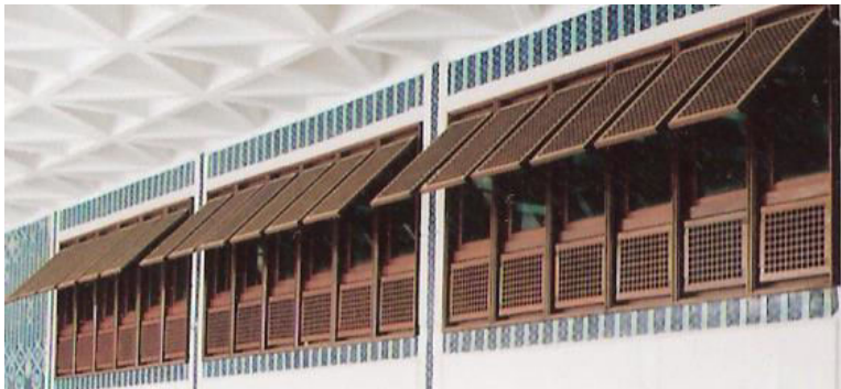
Figure 9. Wooden perforated lattice work used for ventilation in the ablution area.
