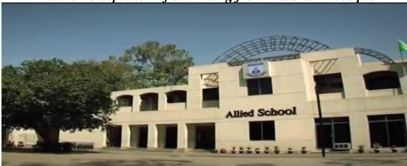
Picture 11 Allied school building
