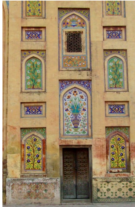
Figure 4: panels of the vestibule from the courtyard side showing Kashi-kari in sunken panels. The middle one is broader and larger panels
