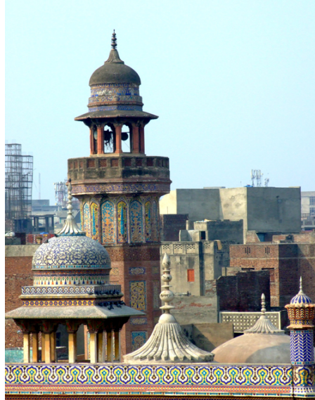
Figure 3: showing in front parapet, and kiosk and in the background minaret
